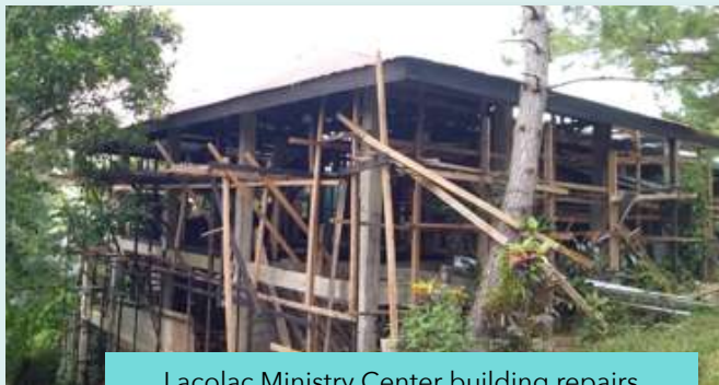
Lacolac Ministry Center building repairs
