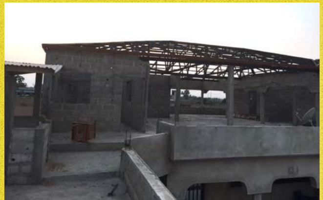
Progress report: house construction
